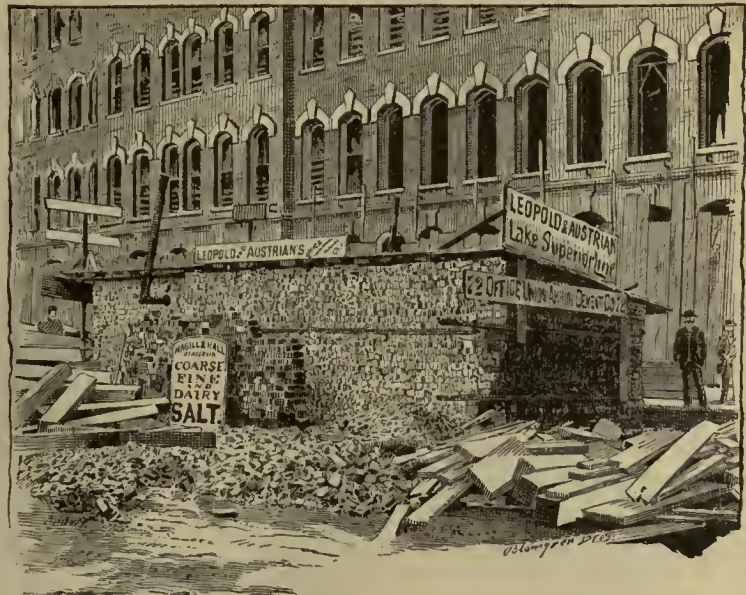
FIRST BRICK STRUCTURE MADE AFTER THE FIRE.
